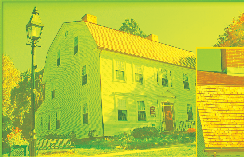
WOOD SHINGLE ROOF WETHERSFIELD, CT
